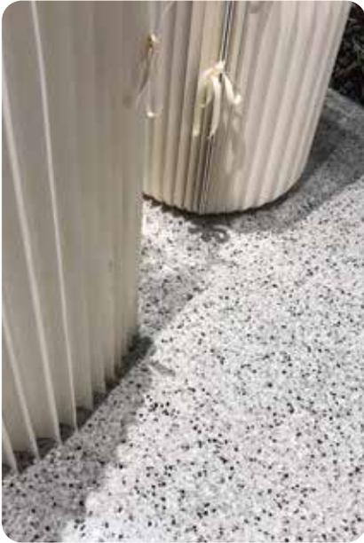
Ready to use just two hours after application, Flowcrete's speediest flooring solution delivers unrivalled installation and cure times as well as an eye-catching finish.
