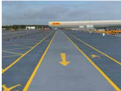
1. Car Park Deck Coatings
